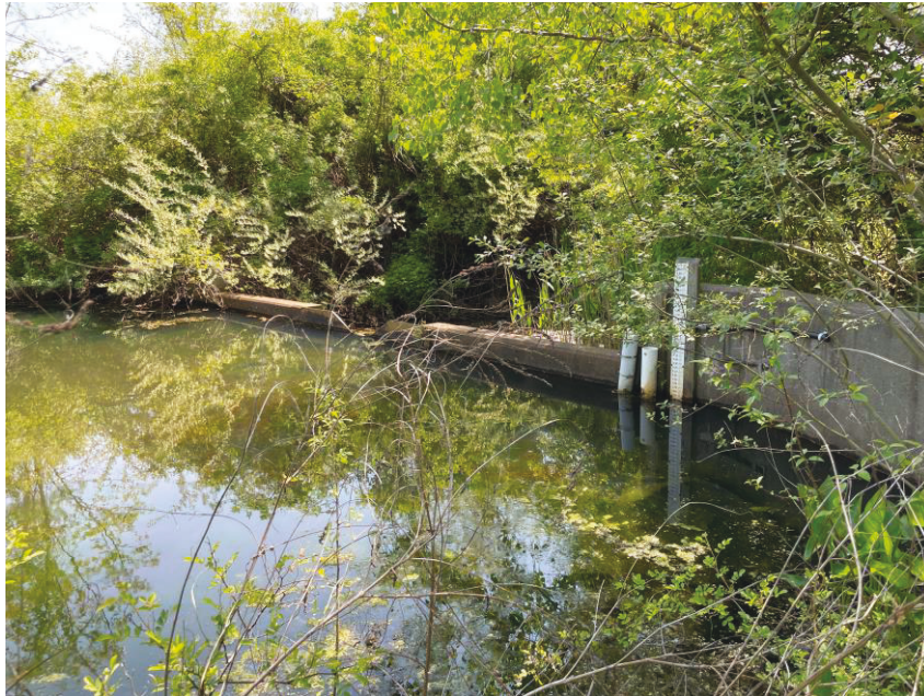
Figure 2: Existing Extended Detention Basin Outlet Weir
