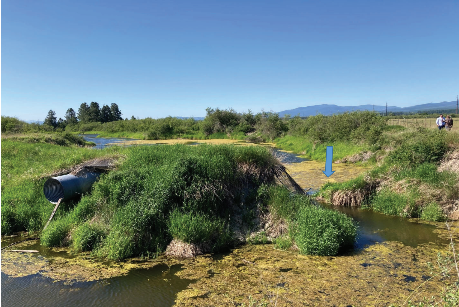
Photograph 5. The Maslonka Dam in Perkins Slough on June 4, 2021. View is generally west by southwest and upstream. The breach in the dam is on the right side of the Photograph (Blue Arrow).
