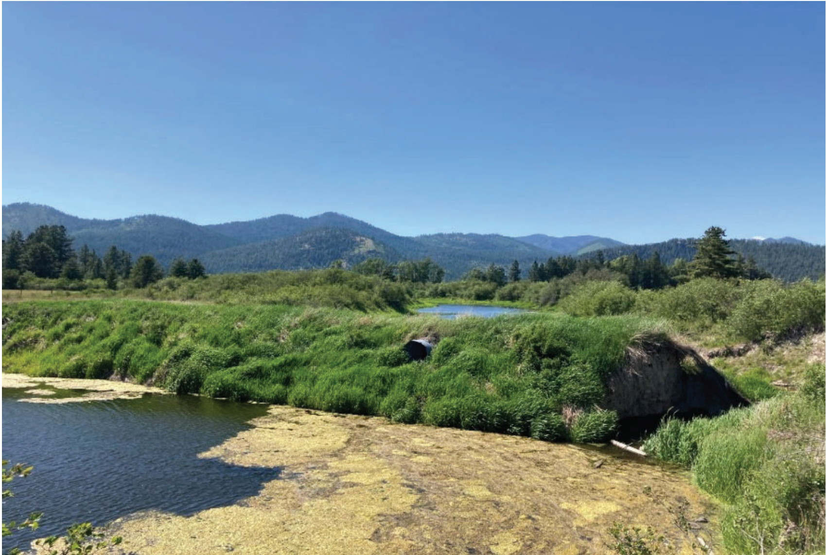
Photograph 4. View of the Maslonka Dam on June 4, 2021. View is northwest and upstream.
