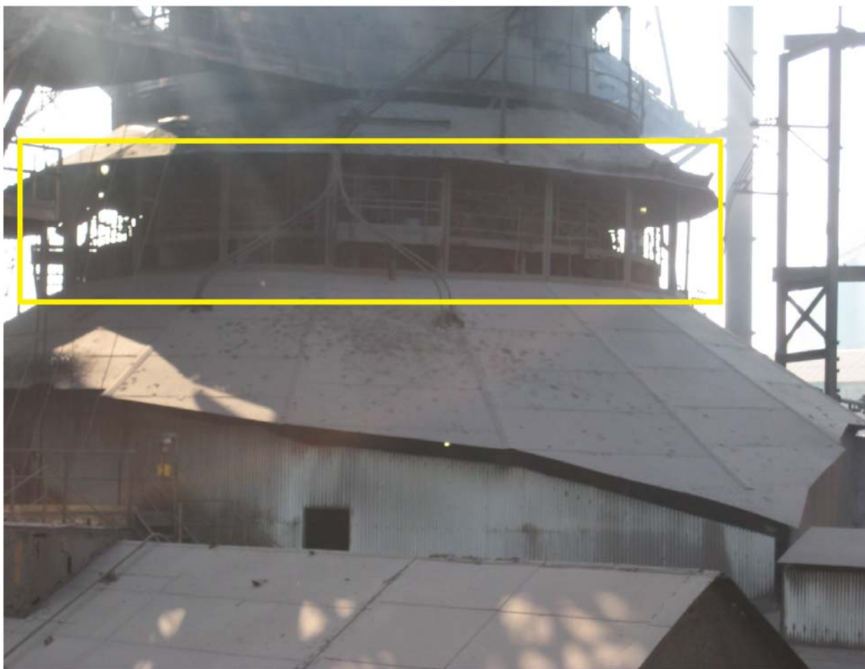
Area to be enclosed in Blast Furnace No. 6 at Gary Works Facility (see Paragraph 13)
