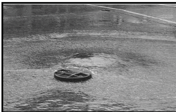
SSOs can include overflows out of manholes onto city streets, sidewalks, and surrounding areas (photo: U.S. EPA).
