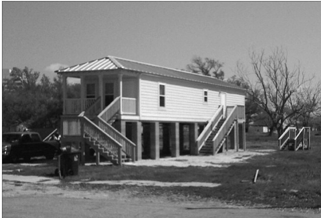
Figure 1. This Mississippi Cottage has been elevated to meet flood elevation requirements.
