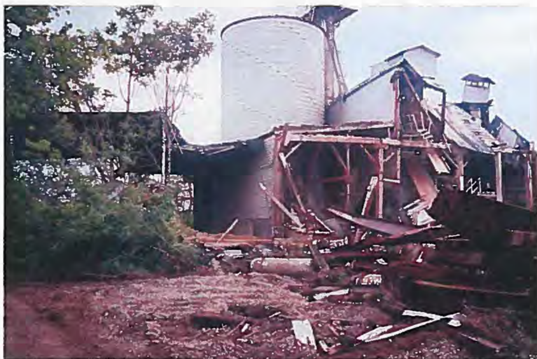
Figure 5 Photo of the demolition of the remaining buildings
