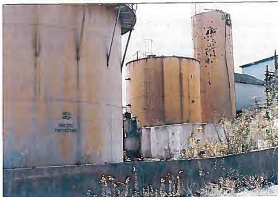
Figure 4 Former Sulfuric Acid Tanks
