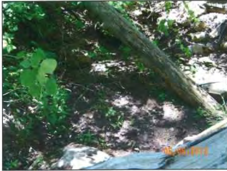
Photo 3. Channel upstream of historical fill at old culvert. Note sediment deposit.
