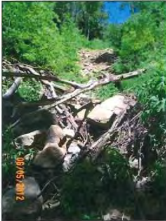
Photo 5. Channel downstream of Chief Portal. Note the abundant woody material.
