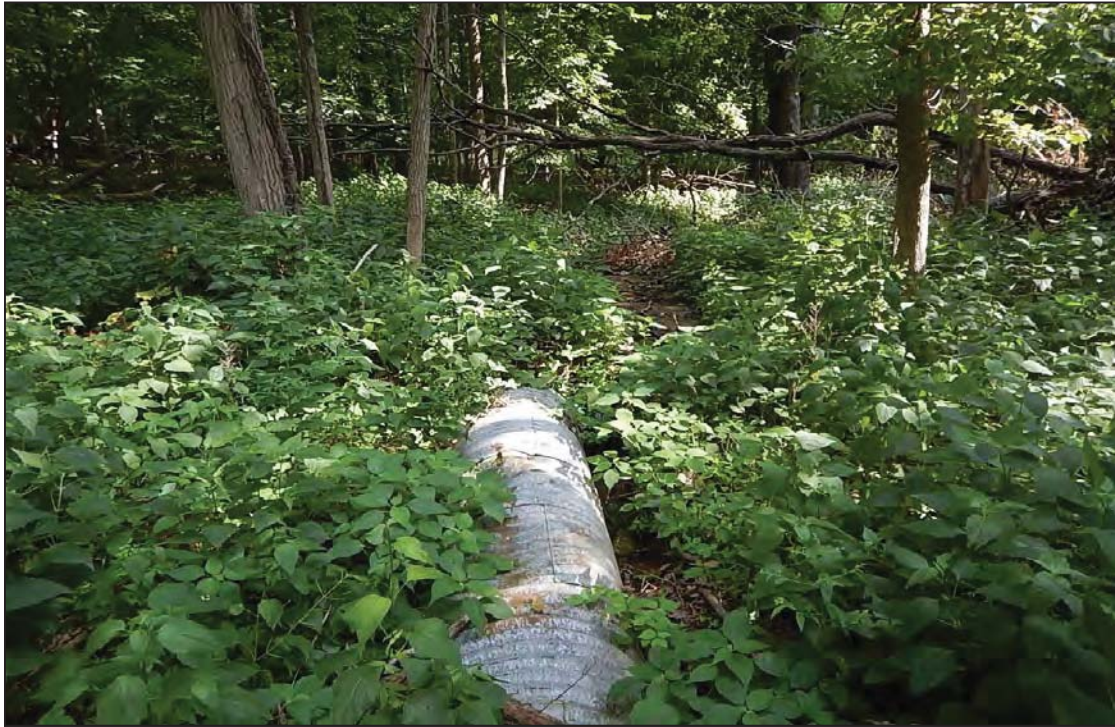
PHOTO 7: Stream 3 looking upstream with culvert in foreground
