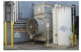
12. Moving the Process #2 King valve will require a complete pump out of the process. Once the valve has been moved and pressure tested, the system shall be recharged and put back online.
